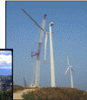
Wind Farm Construction (Unison)
