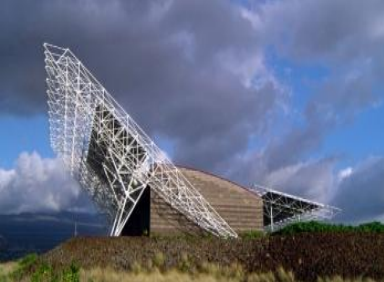
Hawaii Gateway Energy Center
