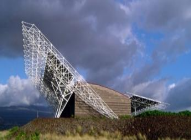
Hawaii Gateway Energy Center
