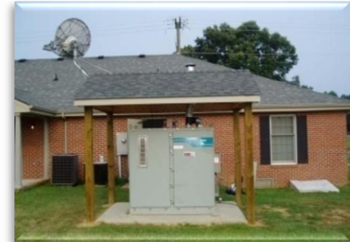
Ida Tech / Fort AP Hill Administrative Support Bldg.
