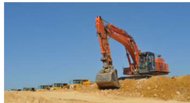
A power shovel removes the first of some 230,000 cubic metres from the Tokamak Pit.
