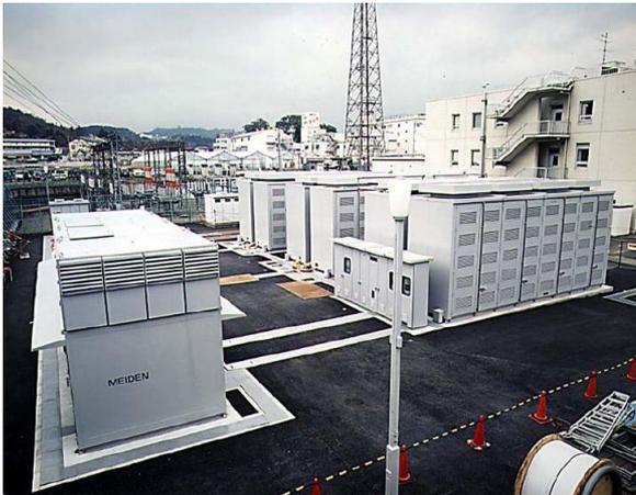
◆ 6 MW (48 MWh) NAS
