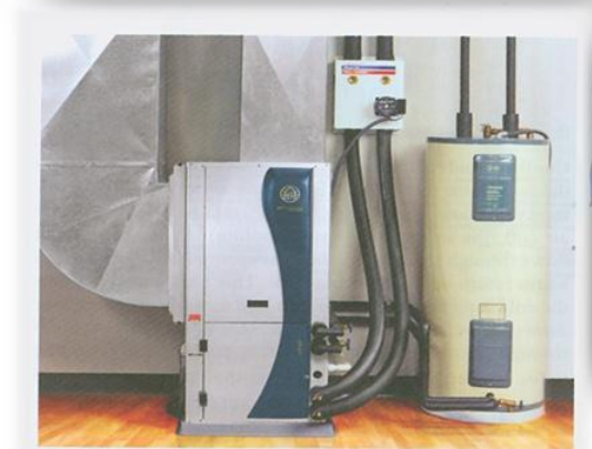
A typical installation of a geothermal heat pump system.
