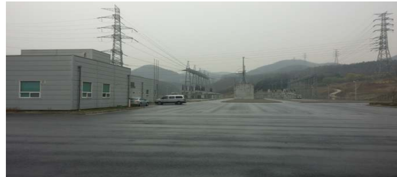
345kV Shin-Yongin S/S (24MW)
