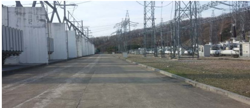
345kV Seo-Anseong S/S (28MW)
