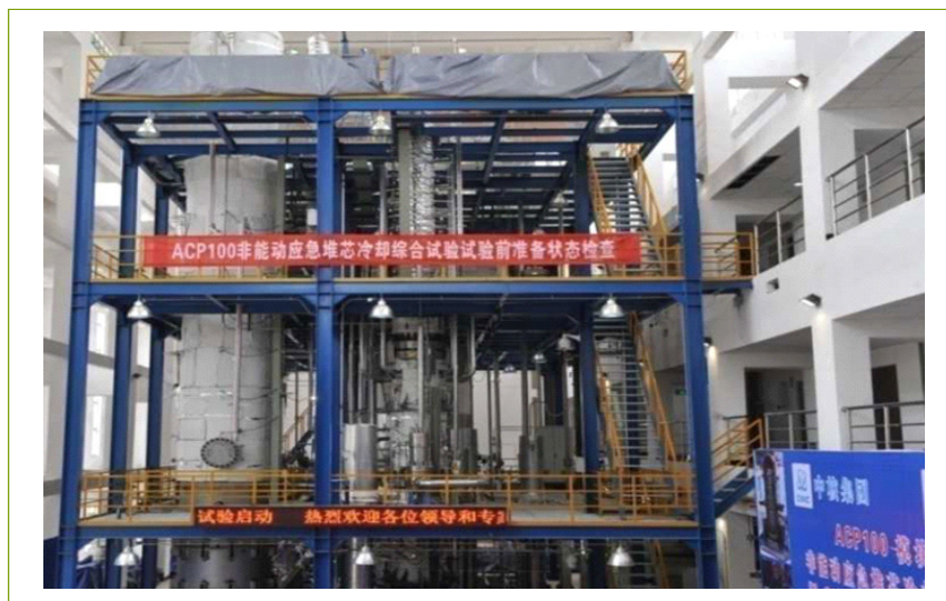
Figure 1 Facility constructed by CNNC to perform core cooling system integration testing and passive residual heat removal system testing for the ACP100.
